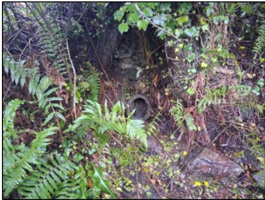
Plate 5-6 Culvert entering the Proposed Development site from the Shannonpark Road.
